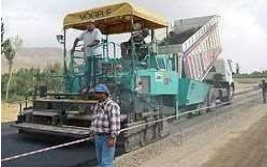
Fig. Road Paver
